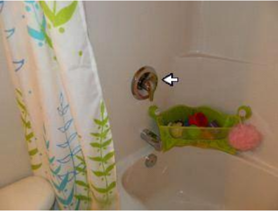
Bathroom Main 4 pc:
